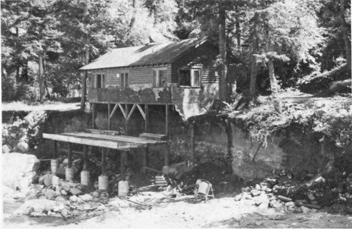
FIGURE 53 Remedial Measures Being Taken for Foundation Repair
